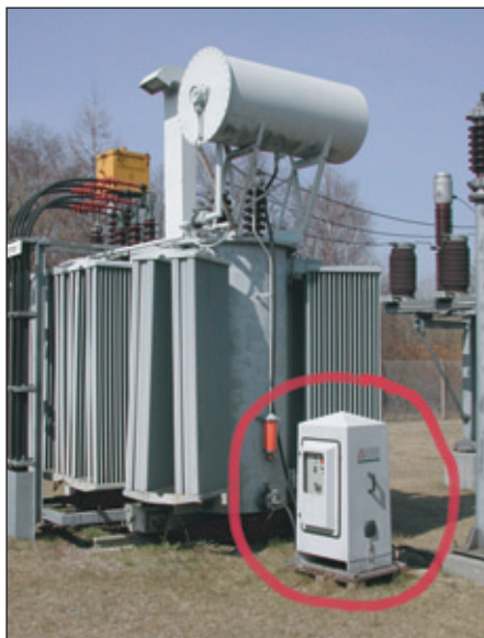
Figure 5. Online dehydration and degassing system in operation
