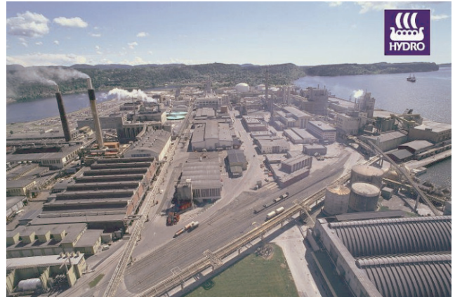
Norsk Hydro Fertilizer Manufacturing Plant
